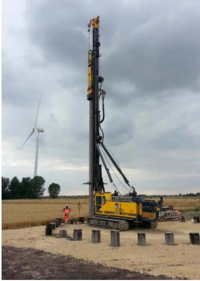
Figure 1. A pile driving rig for pre-cast concrete piles. (Image provided by Anders Beijer-Lundberg)
