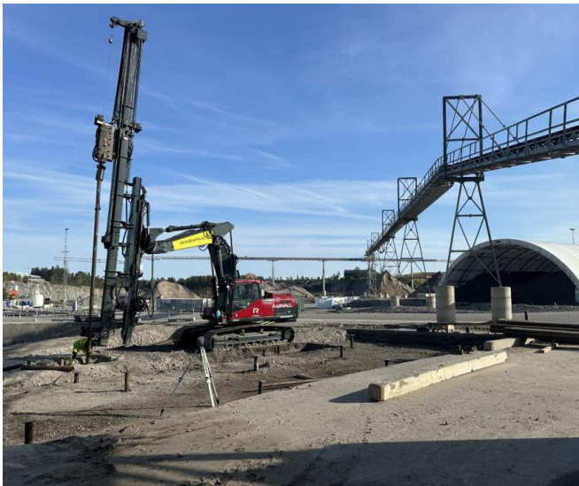
Figure 2. A pile driving rig for driven steel piles. (Image provided by Anders Beijer-Lundberg)
