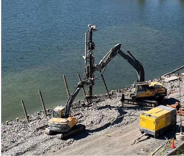
Figure 3. Equipment for drilled piles. (Image provided by Anders Beijer-Lundberg)
